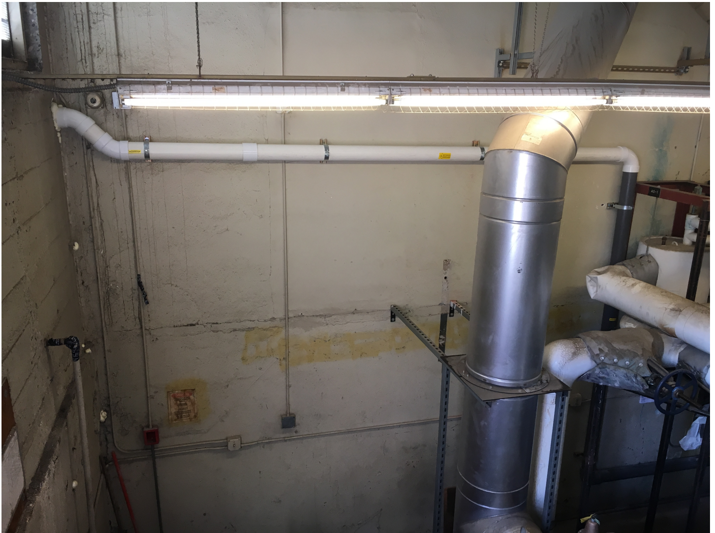
Vent pipe routing to the southern exterior wall in the boiler room. Vent piping was transitioned back to schedule 40 piping when high enough and out of harms way.
