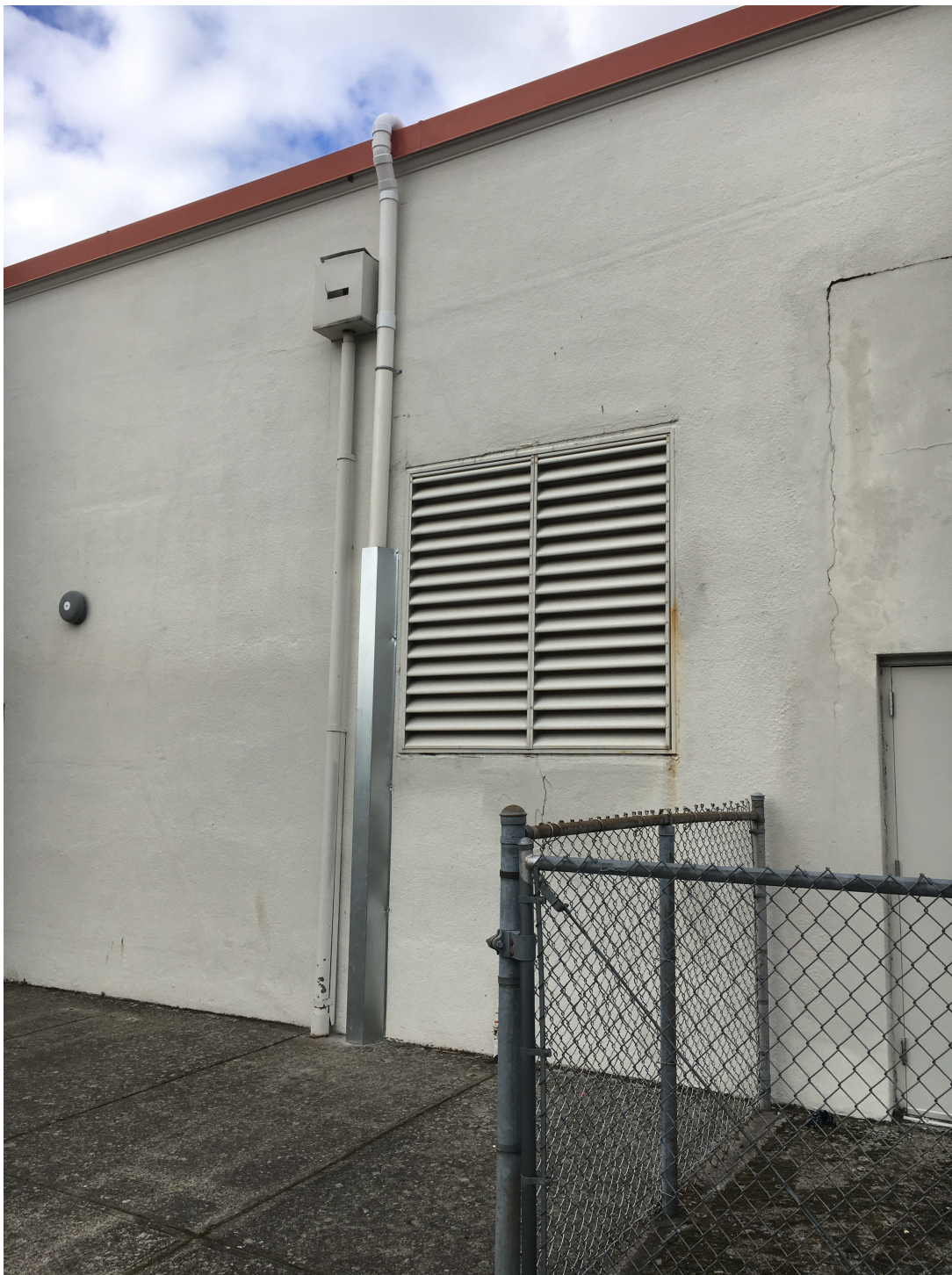
Exterior vent pipe continues up the side of the building and over the parapet wall to the fan location on the roof. The vent pipe was shrouded to deter climbing.
